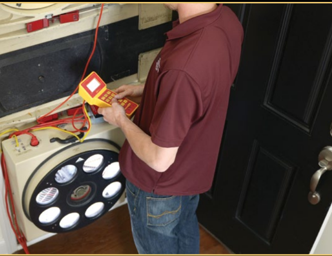
A Blower Door Test is performed on every Schell Brothers Home to obtain your home's HERS score.
