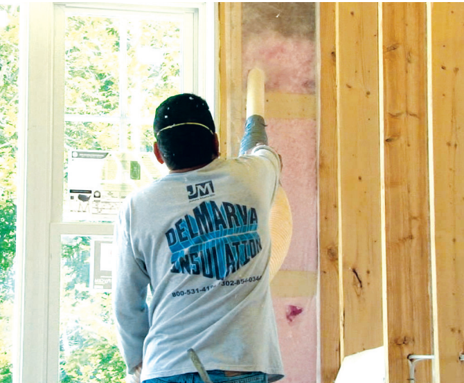
R-23 BLOWN-IN INSULATION
