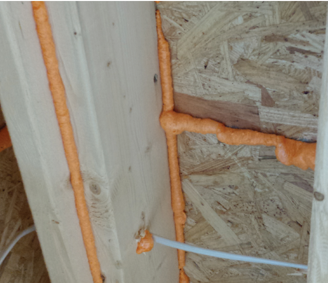
ENERGY STAR DRAFT STOPPING
